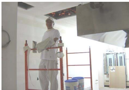
At left, installing door hardware. At right, installing new lighting.
