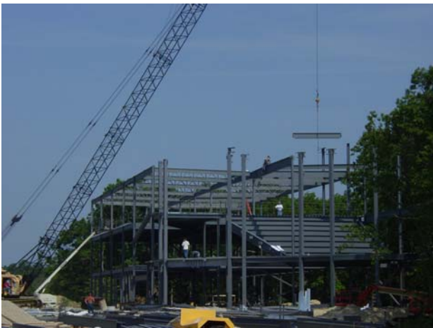
Steel is going up for the north wing lecture hall.
