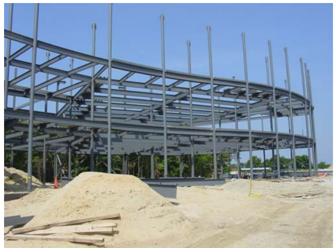
Steel construction of the south wing
