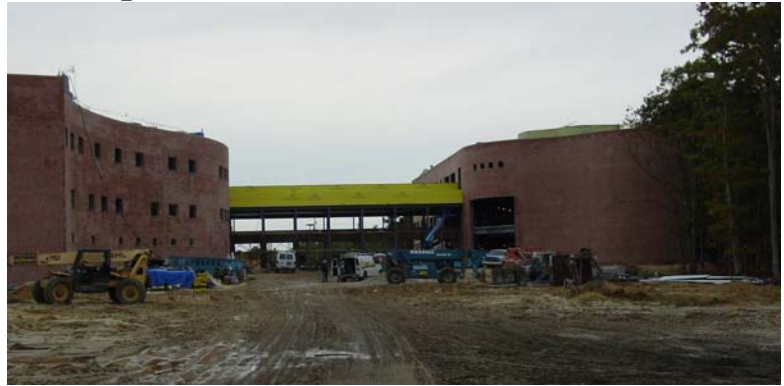
The Cape May County campus project is taking shape.
