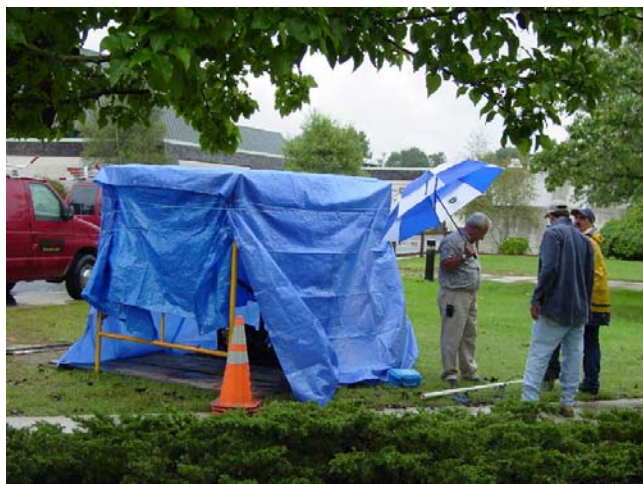
Splicing the cable in the rain.
